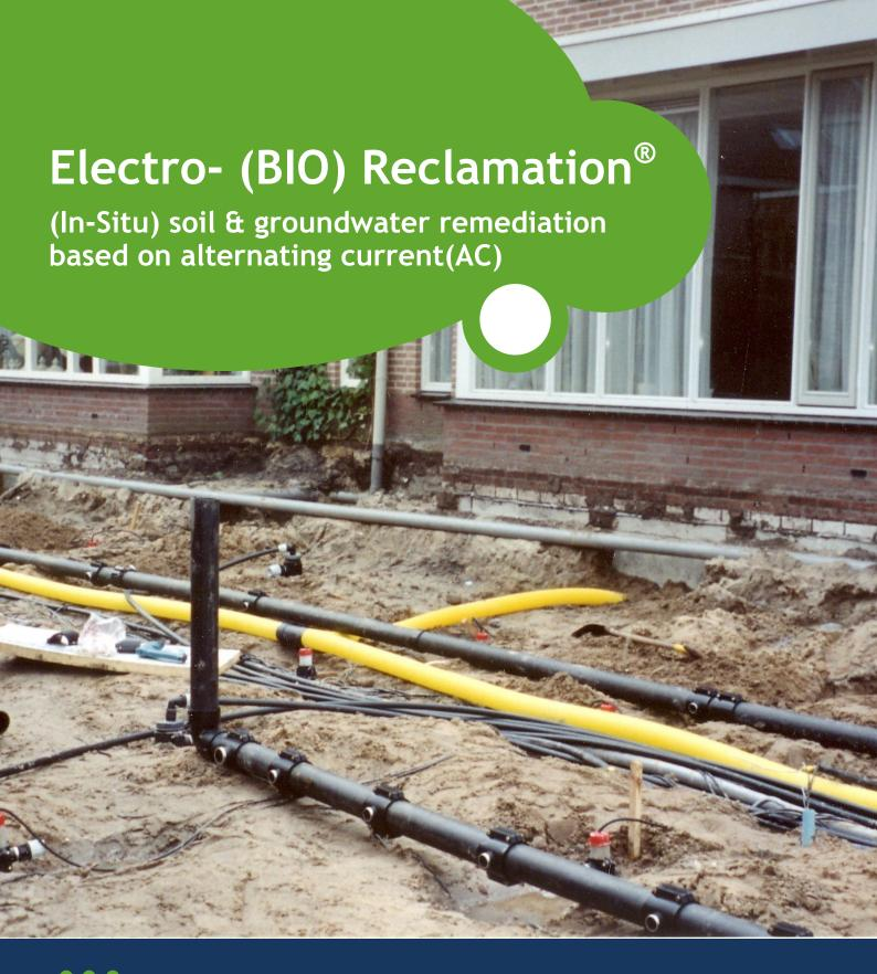
Thermal or thermal/biological remediation of organic contaminations (chlorinated hydrocarbons, aromatics, PAH) in sand, clay, peat or loamy soil. Cleaning the environment with a multidisciplinary approach: heating up the soil in combination with groundwater extraction and increasing the biological degradation as a well accepted and patented technique.
