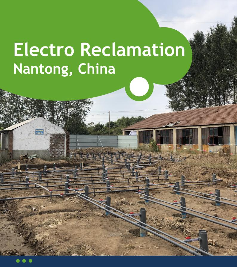
(In-Situ) Soil & groundwater remediation based on Electro Reclamation (ER)
